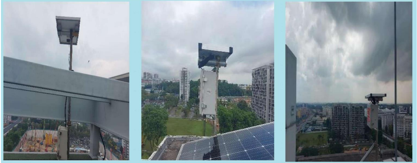
Use of solar panel for construction plant or equipment used on site
